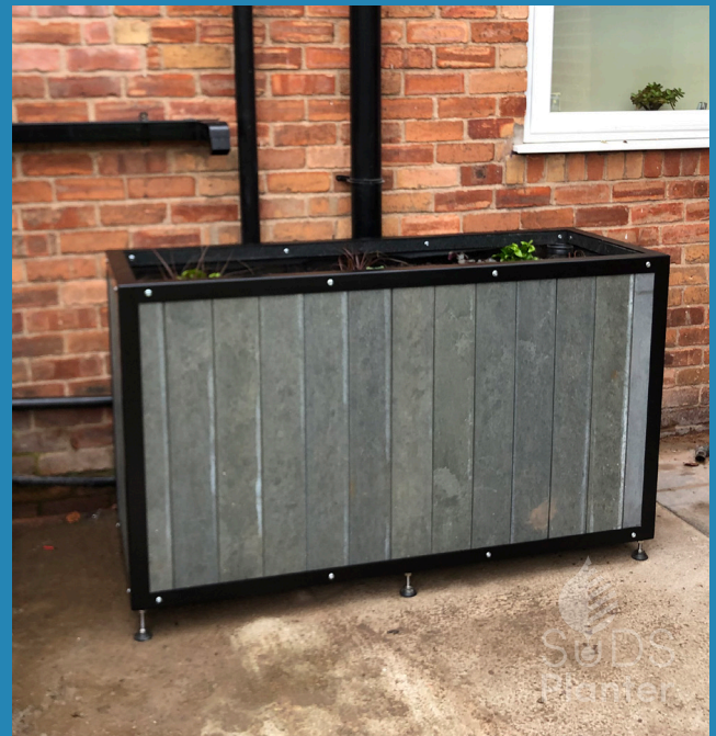
P.2. SuDSPlanter 2 situated against the rear wall and discharging into an existing gully.
