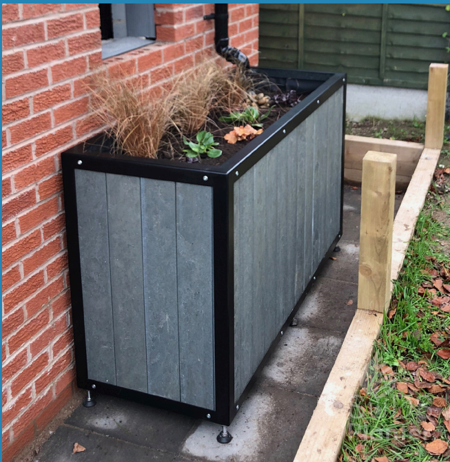
P.1. SuDSPlanter 1 fitted into a tricky location between the extension and a retaining wall.
