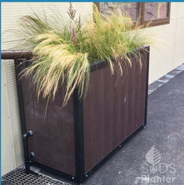
P.1. SuDSPlanter down pipe disconnect drains straight into the surface water sewer cleaning roof water runoff and slowing the flow.
