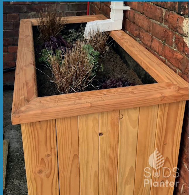
P.2. SuDSPlanter down pipe disconnect of the terraced house downpipe taking approx 25m 2 of roof area discharging to the sewer.
