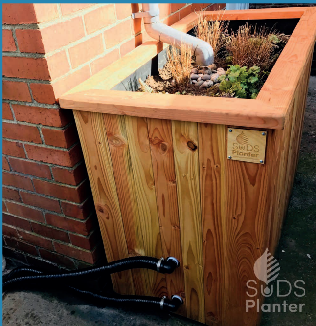
P.1. SuDSPlanter down pipe disconnect of a rear extensions taking approx 10m 2 of roof area discharging to the sewer.
