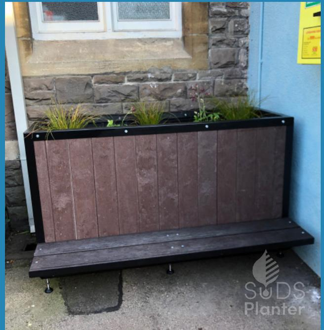
P.2. The centre has installed a SuDSPlanter at the main gate to the community centre, forming an entrance feature and addressing surface water flooding downstream.
